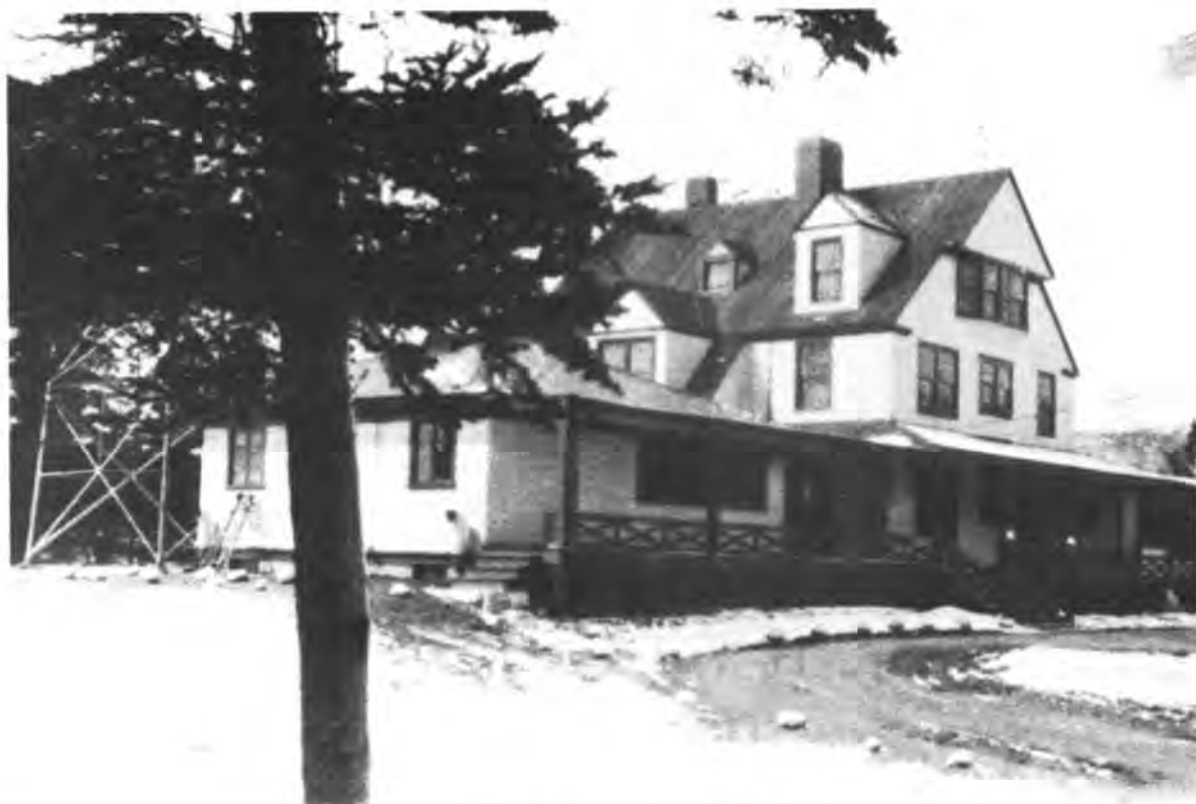
The Bar Harbor Country Club building leased by Mr. Fabbri for use as NBD control and receiver station. Photo courtesy Carl Herr.
